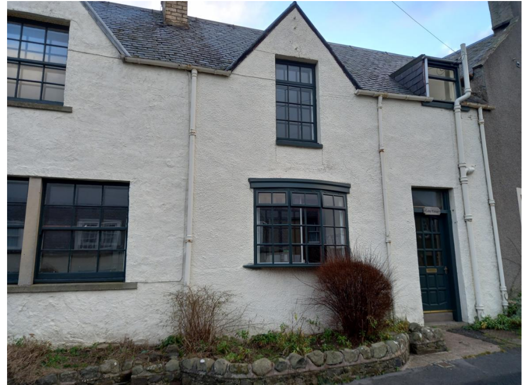
Figure 5: Original Windows and Door
