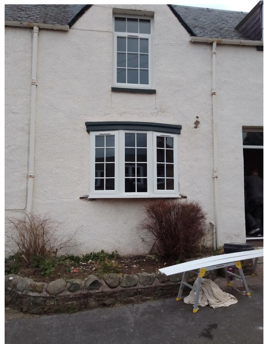
Figure 6: Image of Replacement Windows
