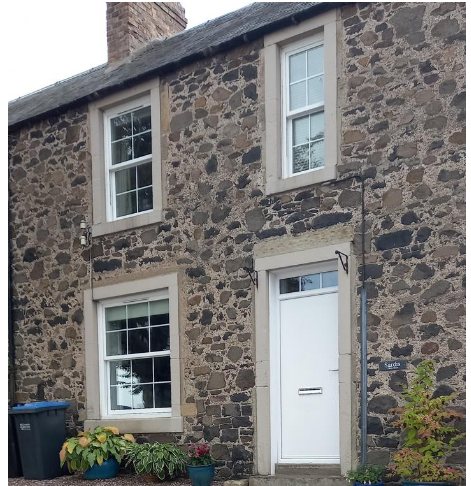
Figure 10: Image 1 of nearby property with uPVC casement windows at Sardis, Main Street, Morebattle.
